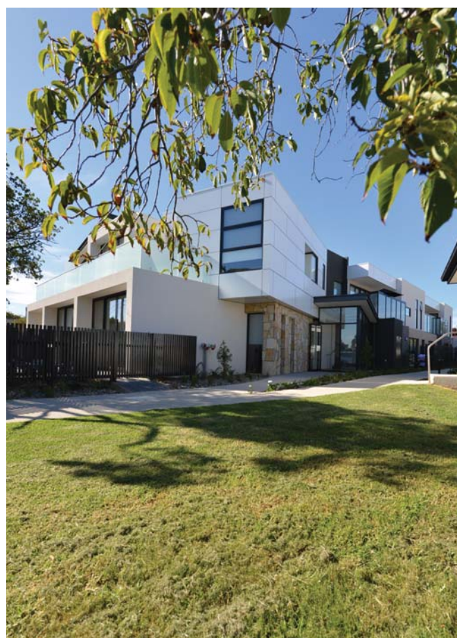
Pictured: New Mentone affordable housing units.
