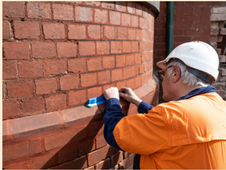
Brick restoration work continues
